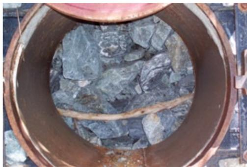
A single stick can cause a culvert to plug.
