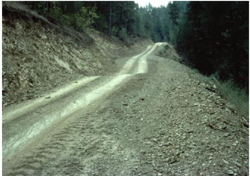
*Rolling dips are highly effective road drainage structures.*
