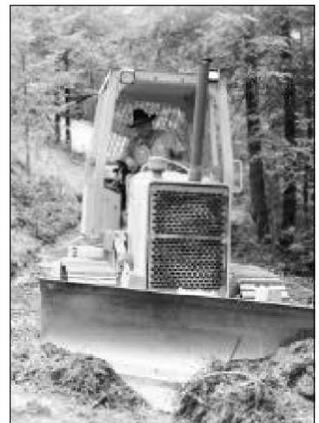
*Forest management requires diverse skills. Here Jim Doerksen is working on road rehabilitation, knocking off the outside berm to allow water to drain. Some sections of the road have been rocked for erosion control.*
